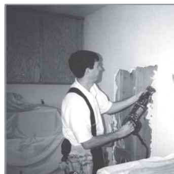
Mr. Christian Nelson cuts a hole in the wall to create a new entrance for the office.
